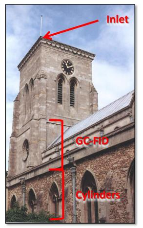
The project involves installing 4 Ellutia GC machines in the East Anglia region to measure atmospheric methane concentrations. We install the machines in church towers to minimise strong local fluxes being recorded and to ensure more regional concentrations of methane are measured.
